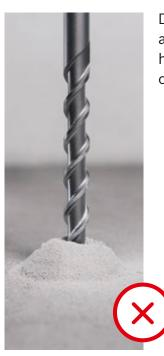
Dust remains in and around the drill hole after drilling is complete
