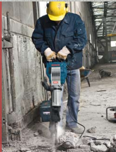
Chiselling performance in concrete C 30/35
