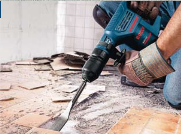
Material removal rate – SDS-plus tile chisel
