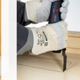
Trimming and correcting work
