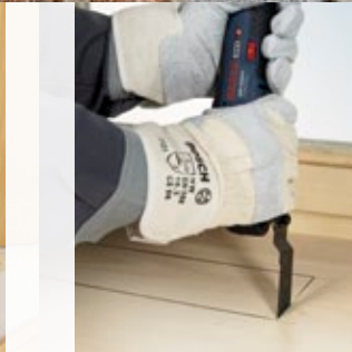
Trimming and correcting work
