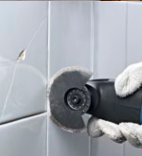
Tile or bathroom renovation
